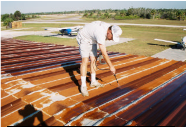
Hanger Roof Repairs by Jerry Grondyke
